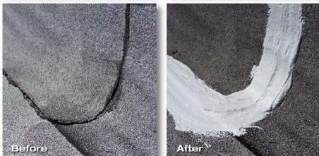
New and improved technology allows for GacoPatch to be the long term solution for roof repairs. It does not contain asphalts or acrylics and it is extremely durable. GacoPatch remains permanently flexible even under permanent ponding water. It is UV stable and will not chalk, crack or peel. No reinforcements or extra steps are required for horizontal patches, even over 1/2" thick, because GacoPatch resists degradation over time and will not become brittle or break down.
